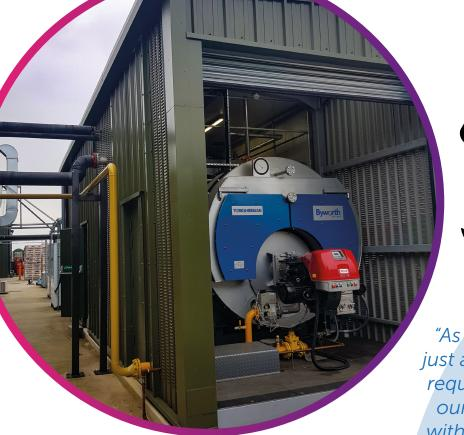
As a result, the 3500kg/hr boiler was subsequently replaced with a larger, tailor-made 4500kg/hr unit under a renewed 12-month hire contract, enabling the company to meet its growing order requirements.
